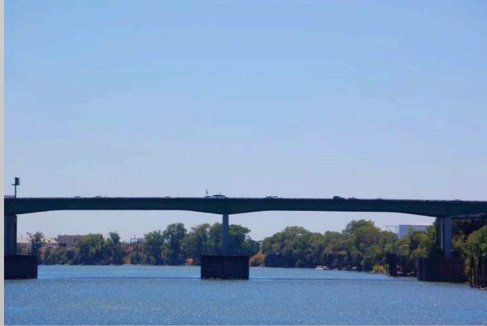
PIONEER BRIDGE (1971) Sacramento
