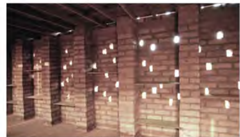
Sra Pou, Cambogia- Rudanko e Kankunen Architects
