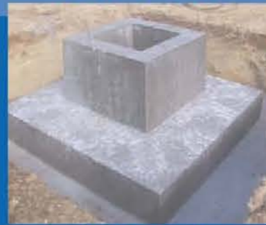
reinforced prefabricated concrete pierth
